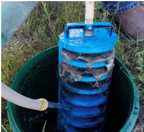
Remove the filter from the outlet T-baffle sleeve & wash over the inlet riser.
