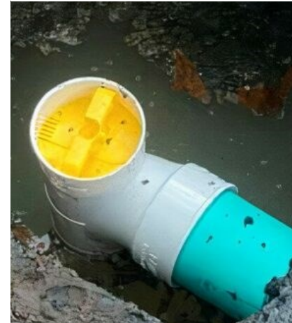
Replace filter into the T baffle with the arrow pointing out.
